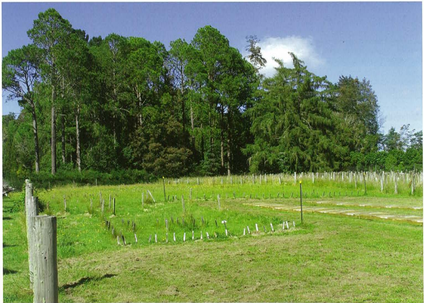
Far left and above: Field test site located at Whakarewarewa, Scion, Rotorua. Far right: Service test for a locally grown western red cedar building with split shakes on the roof and gable ends
