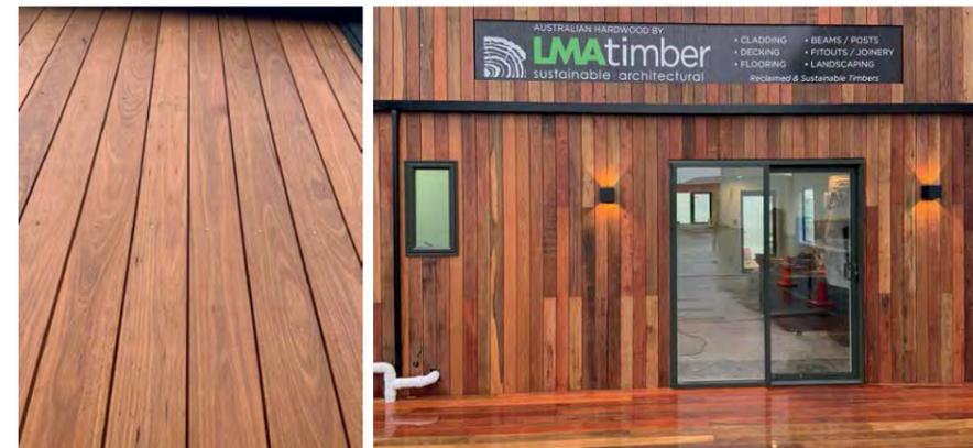
Clockwise from top: Grey Ironbark decking has decades of natural durability; the new LMA Timber showroom under construction; cladding can be supplied oiled and dressed or left for customers to finish.
